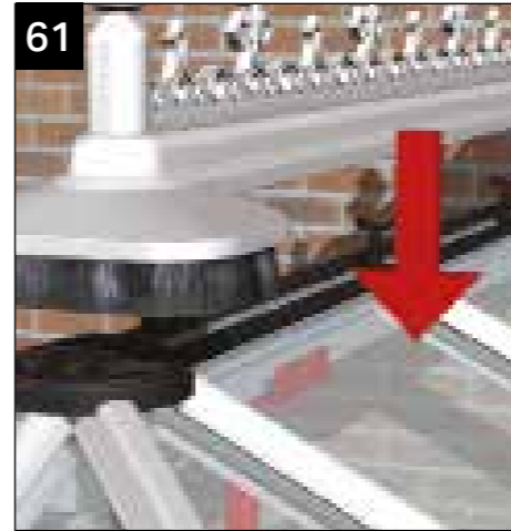
61 Offer up the complete ridge capping onto the roof.
