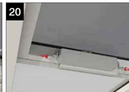
20 Fit provided securing bolts into the motor body through the location holes in the brackets.
