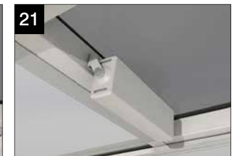
21 Finished mounted motor in situ. Note: For further details, refer to motor instruction guide which can be located in the motor box.
