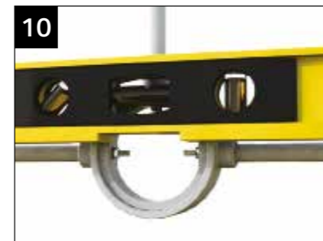
10 Now, finally check that the horizontal elements are level and the vertical element is plumb. CHECK THAT THE SIDE FRAMES ARE STILL PLUMB. Spanner tighten the boss nyloc nuts.
