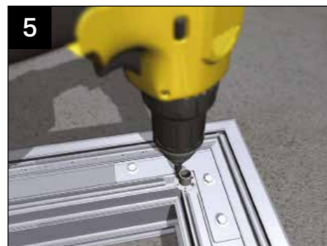
If supplied, fasten to each corner the tie bar drop rod fixing bracket to the underside of the lantern eaves beam.
