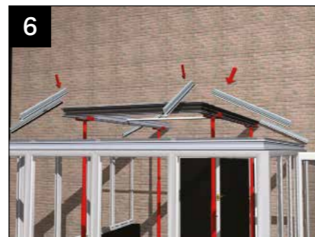
Now the Lantern eaves beam is assembled into a one piece structure, temporarily support it. Attach the glazing bars according to the component location plan. Tighten the bars, at the pagoda beam end first and then at the main eaves beam second.
