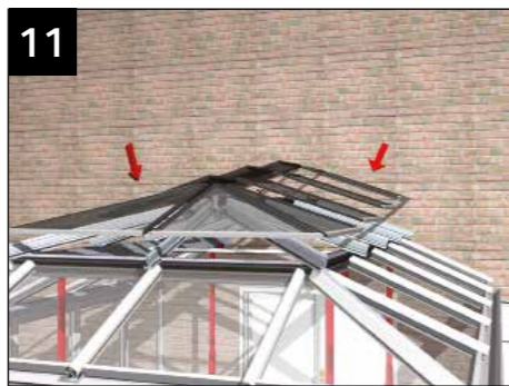
11 Glaze the upper pagoda roof, and complete all external works
