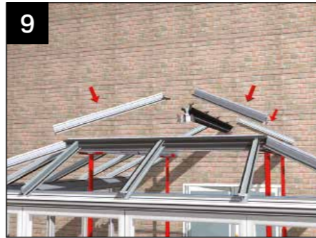
9 Using the roof location plan, build the upper roof as per section 4 of this guide.
