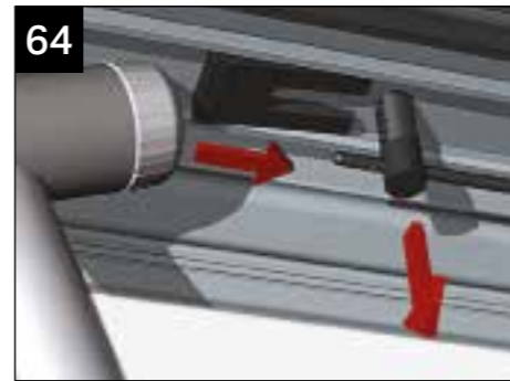
64 Pull down on the T bolt and tap the fixing wedge into place to secure the T bolt. Cut off the excess T bolt below the fixing wedge.
