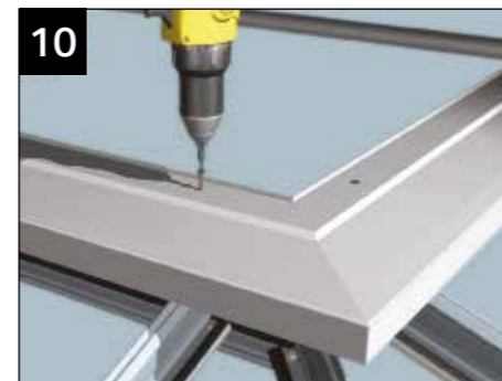
For the lantern application, attach the PVCu window cill to the beam. Assemble side frames on to pvc cill and build the lantern roof as per section 4 of this guide.
