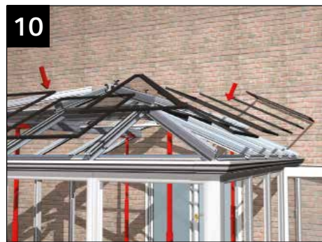
10 Glaze the lower pagoda roof fully.
